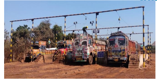
Tarpaulin covering facility for loaded trucks
