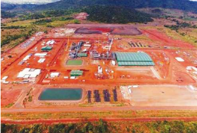
Balama Graphite Mine in Mozambique
