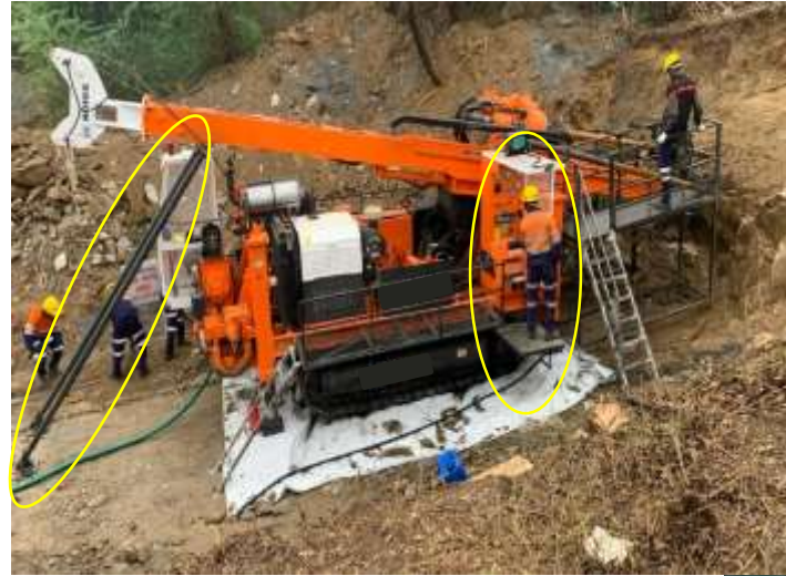
Shallow Angle Drill Rig
