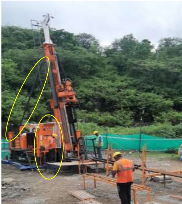
Conventional Drill Rig
