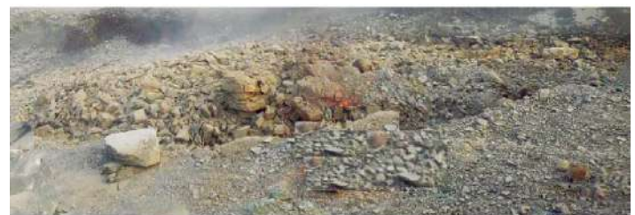
Blast performance with stemming plug
