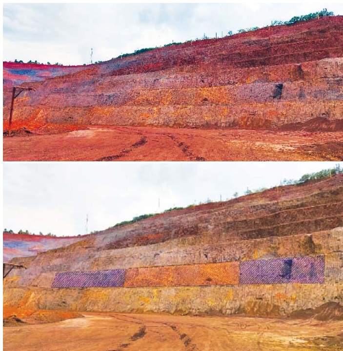
Fig. 3.3—SLO with limonite bands are marked in the red zone, while SLO with powdery ore are marked in the blue zone.
