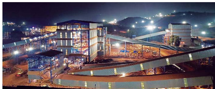
Fig. 1.1 – Central Processing Unit (CPU) at Nuagaon Iron Ore Mines of JSW Steel Limited
